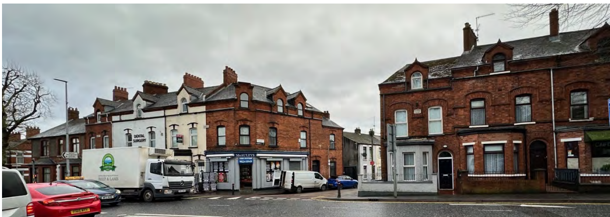
Figure 1. A recent view of Glenalina Terrace (left) and part of Clondara Terrace (right) on the Falls Road. Eileen was born above the corner shop (now 424 Falls Road, McAuleys butcher's) which in 1913 was run by her father as a spirit grocer. The brown door at the right is the entrance to 2 Clondara Terrace (now 428 Falls Road) where her grandfather and several of his children lived. The family home of James Connolly was at 420 Falls Road; it is now a dental surgery. (Credit: Carl Murray)
